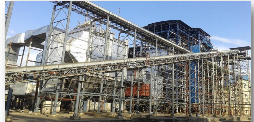
BAGASSE HANDLING SYSTEM
