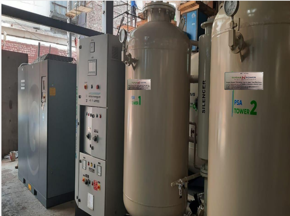
OXYGEN PLANT (PSA TOWERS)
