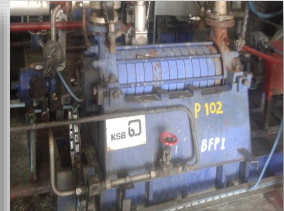
BOILER FEED PUMP
